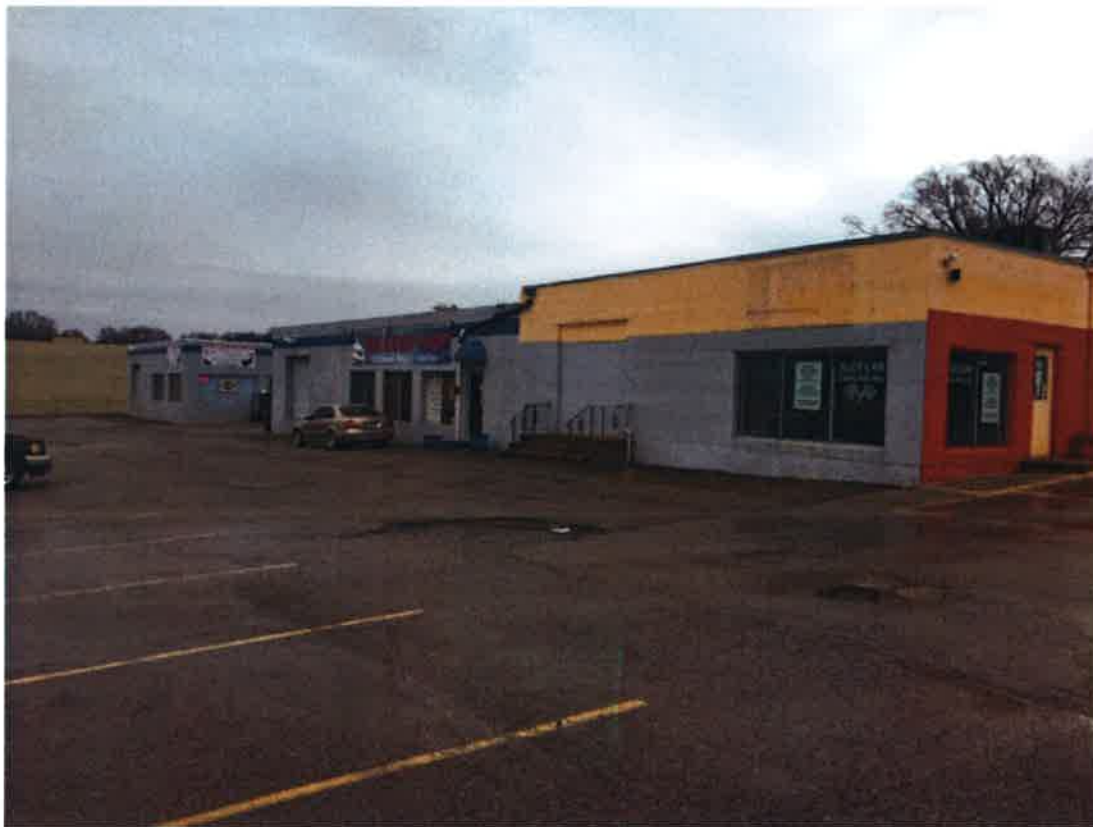
Figure 2. Front View of Building. Kandy Shop is Middle Tenant.
