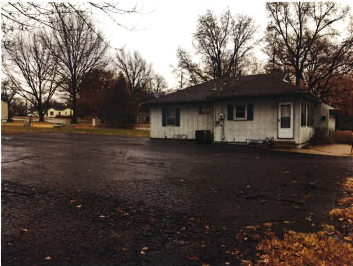
Figure 3. Parking and Dropoff area on West Side of Building
